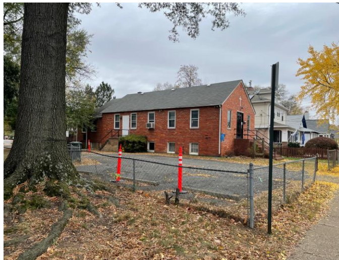
Figure 2: Photograph of site
