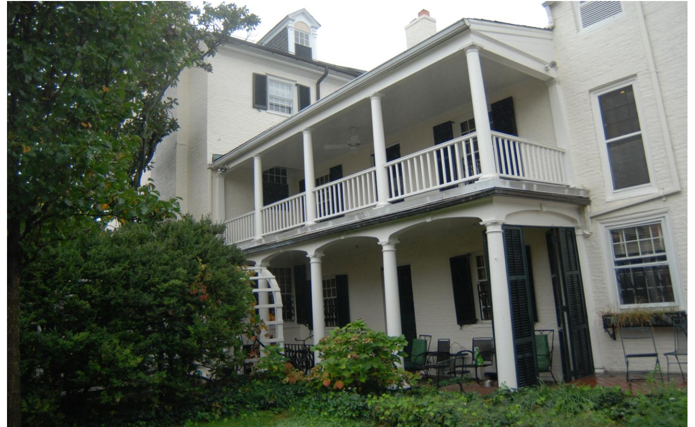
East Elevation of EII looking Southeast towards main block
