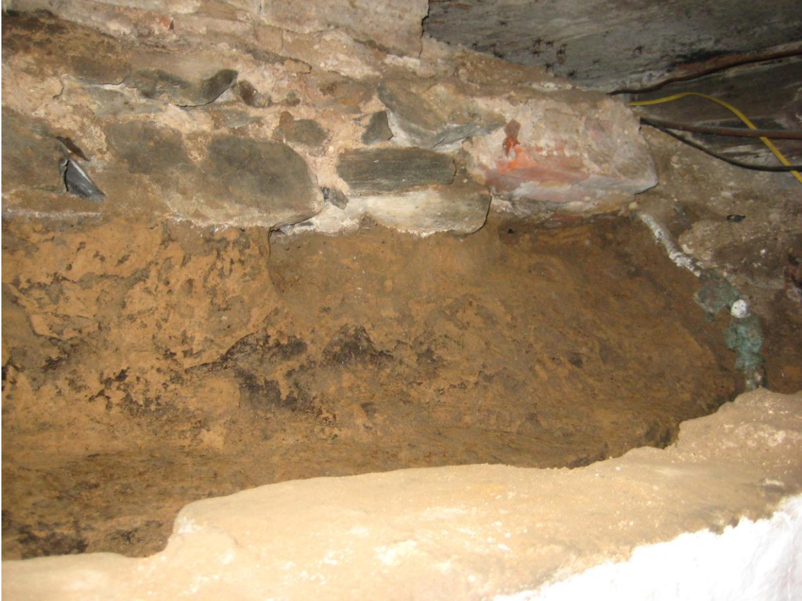
Figure 5. Detail of the bottom courses of the stone base for the fireplace and the terminus of the brick arch. The base is laid on the natural clay subsoil, which slopes down to the level of the cellar builder's trench.
