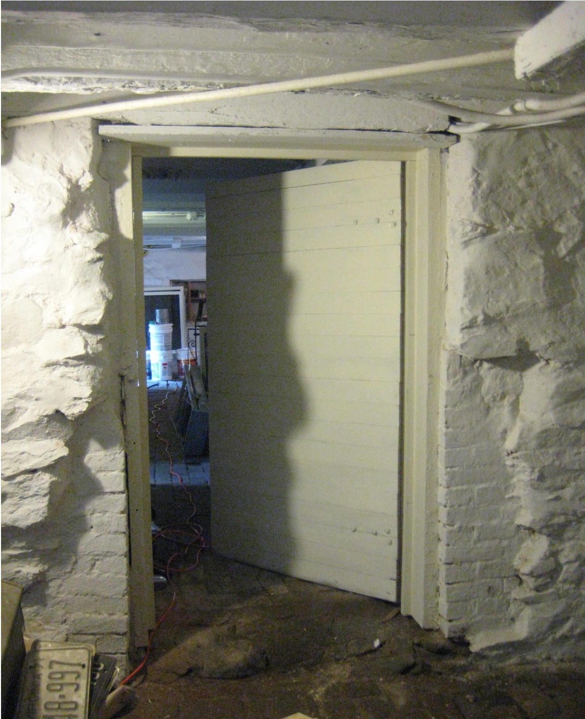
Figure 2. Detail of the doorway in the south foundation. Note the relatively irregular character of the stonework and the brick infill on either side of the doorway.
