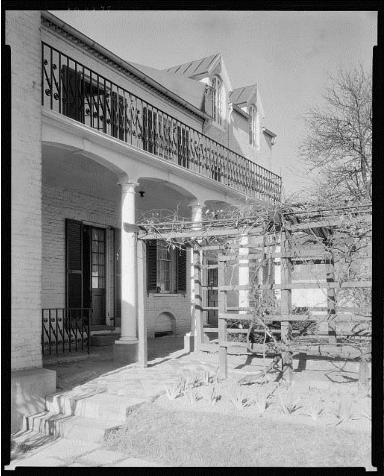
Figure 4: East elevation of the rear ell, circa 1930-39, showing alterations likely made by Gay Montague Moore. Image source: Library of Congress Prints and Photographs Division. http://www.loc.gov/pictures/item/csas200906956/ .
