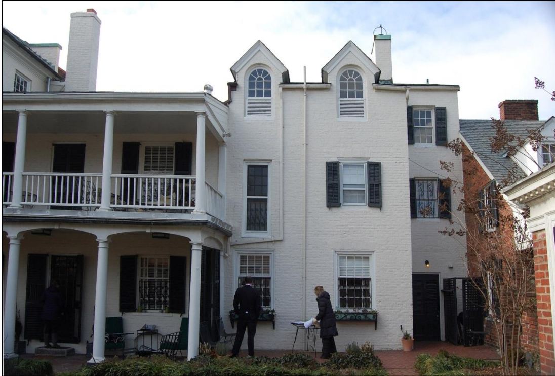
Figure 5: Portion of the east elevation at the first floor that is proposed for demolition and capsulation for the kitchen addition
