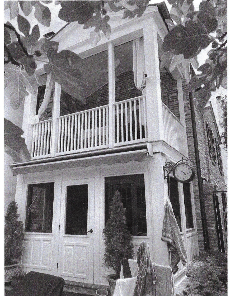
SCREENED PORCH - SOUTHWEST ELEV.
