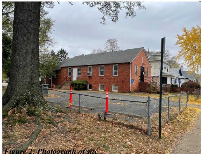
Figure 2: Photograph of site
