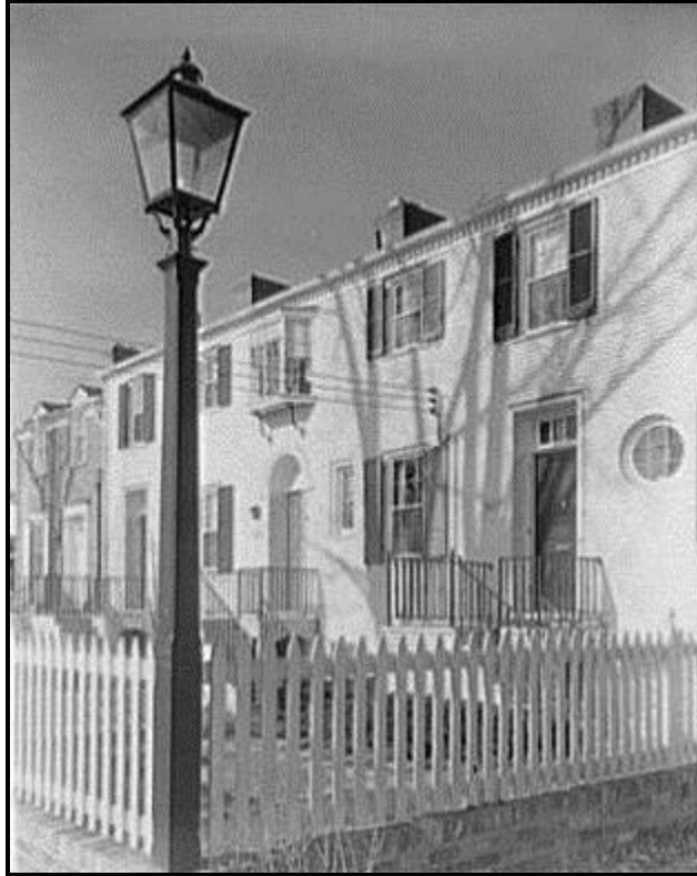
Figure 2: Library of Congress Photo of Mid-20 th century Yates Garden Townhouses
