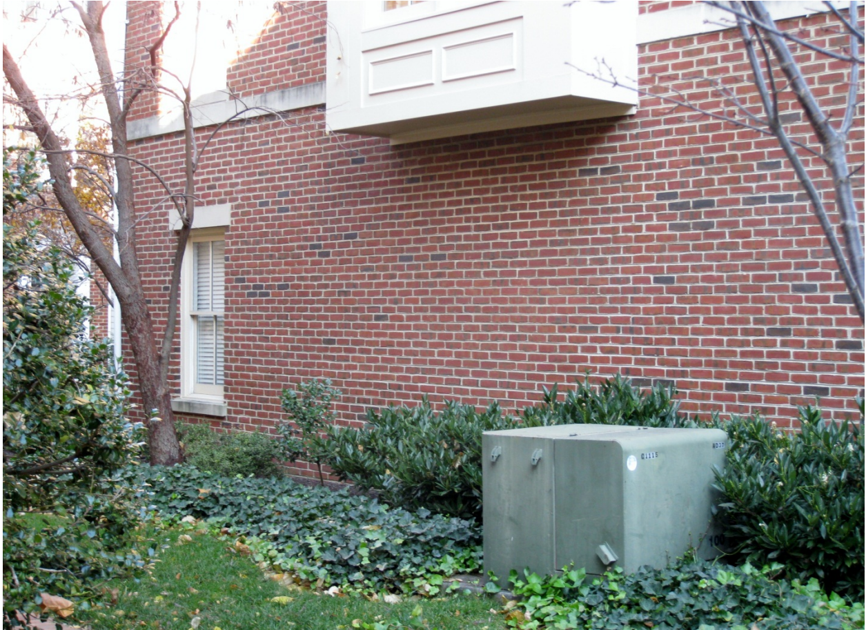
Figure 11: Category VI – Ground level installation below bay window.
