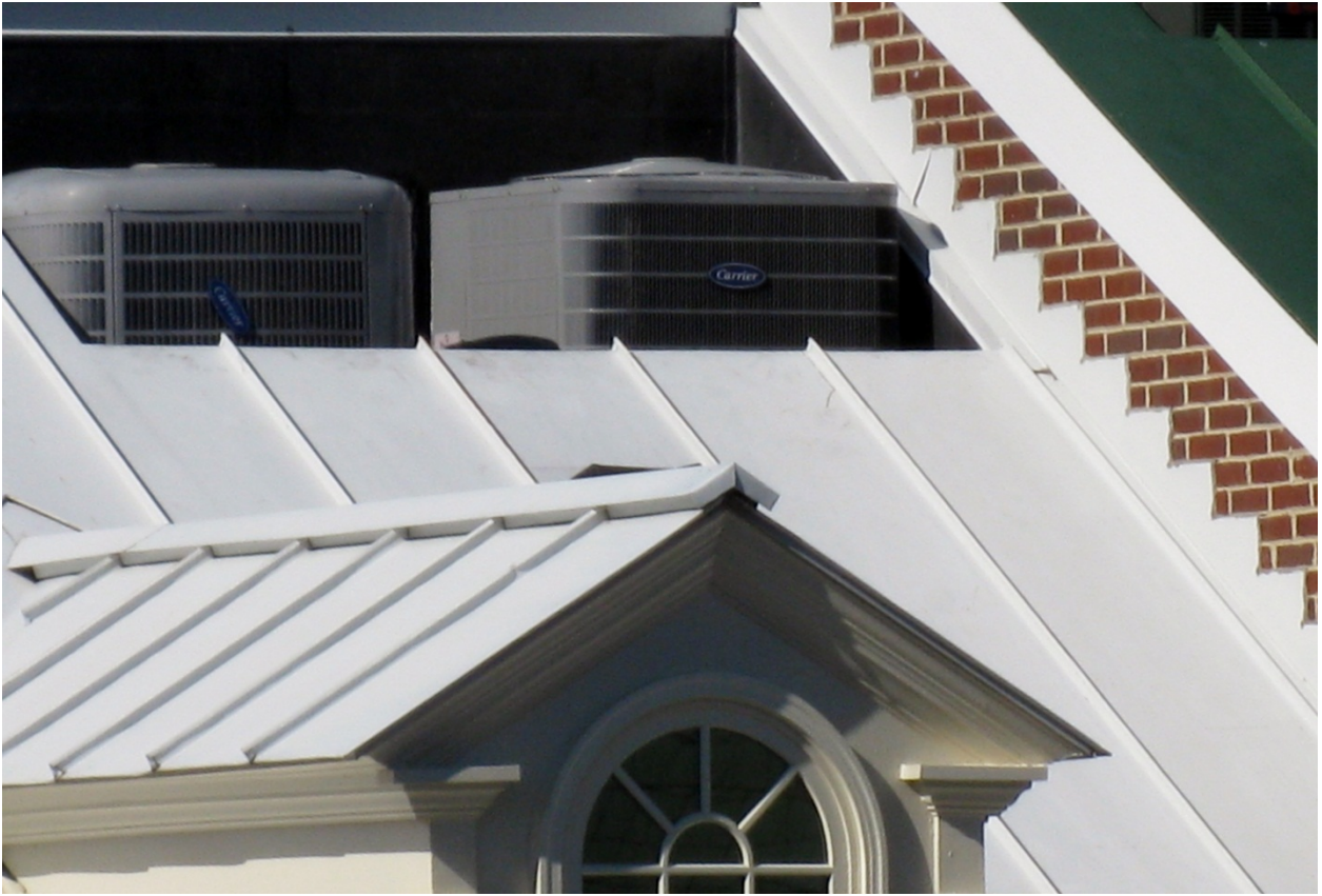
Figure 7: Roof cut-out installation.
