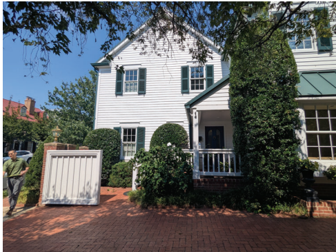
View Of Existing Entry Porch & Door
