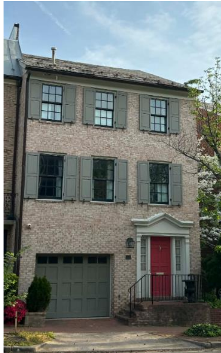
Figure 1. View of the subject property’s roof from Queen Street.
