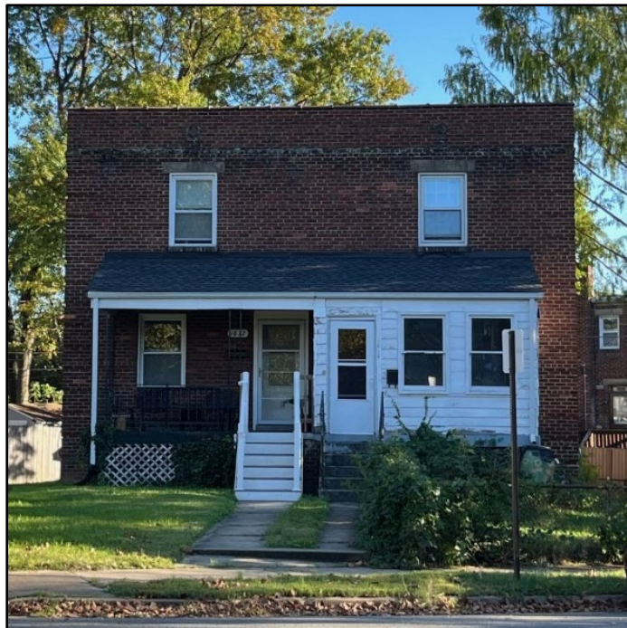
Photo 1: Existing conditions at 1612 & 1614 Princess St.
