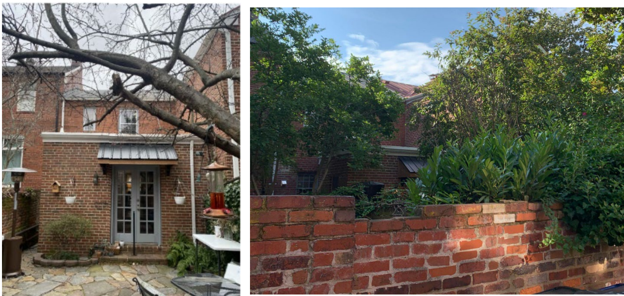
Figure 1. Existing one-story rear addition viewed from backyard (left) and public alley (right).
