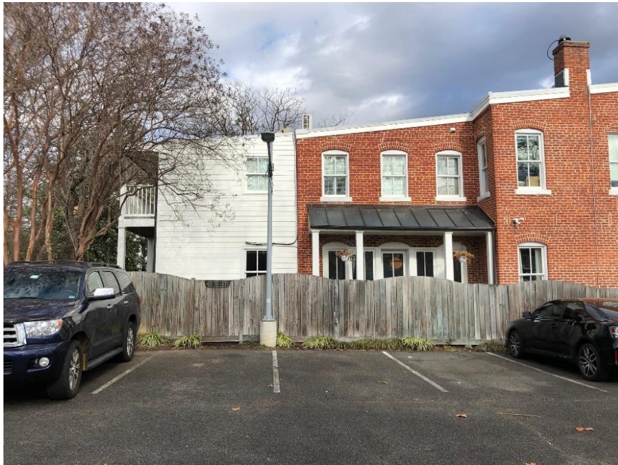
Figure 1: Existing north light
