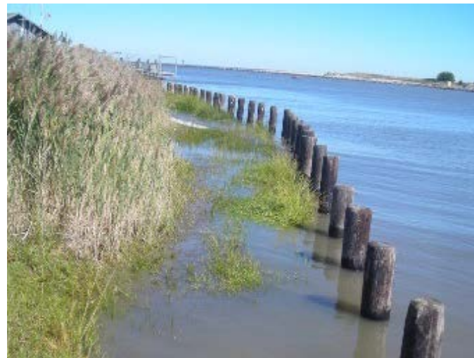
Bulkhead/Living Shoreline Hybrid
