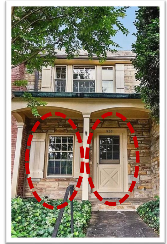
903 S. ST. ASAPH ST. OPERABLE WINDOW DIVIDED LITE FRONT DOOR
