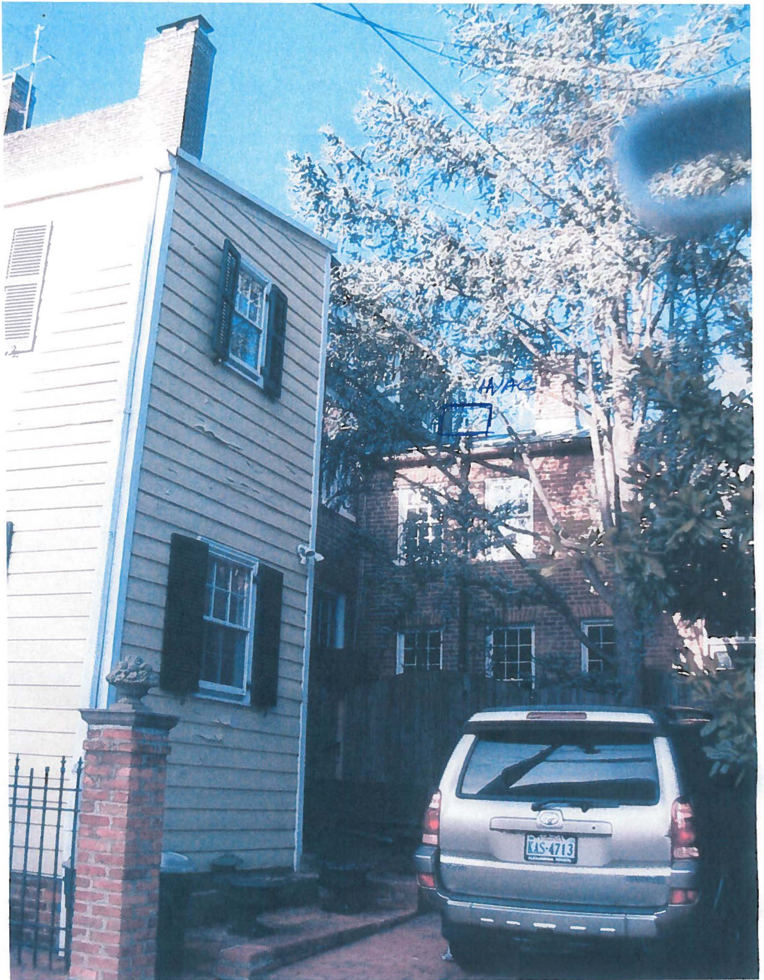
BACK FACADE - 203 CAMERON ST. - L WING ROOFLINE
