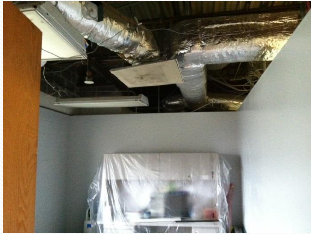
Insulating ductwork to Administration Office.
