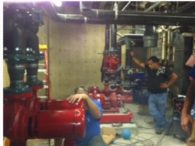
Connecting new pumps to new boilers.
