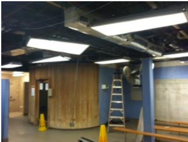
Fan coil refrigerant lines and pipe insulation work.
