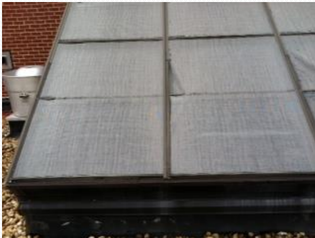
Skylight-screens ready to be removed.
