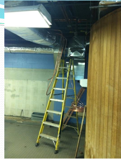
Refrigeration lines installation and new ductwork at Locker Room
