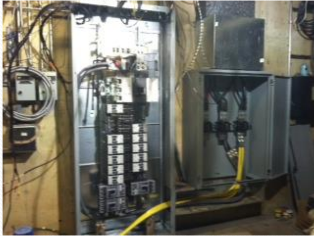
New electrical switchgear system.
