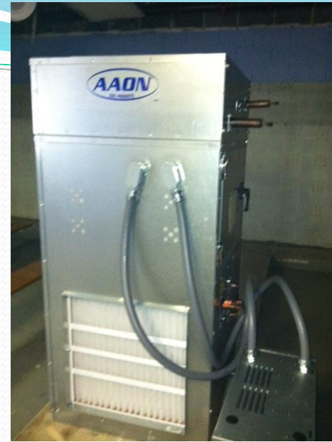
New Aaon air-handlers to serve locker rooms (one of two).
