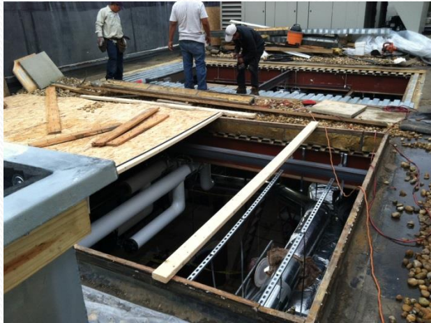
Insulating new ERUs and RTU #3 curbs.
