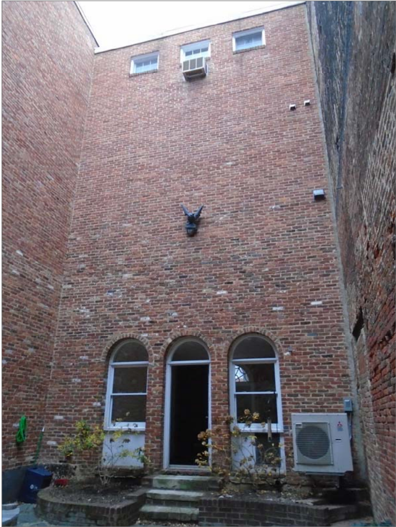
EXISTING REAR ELEVATION - FULL WALL
