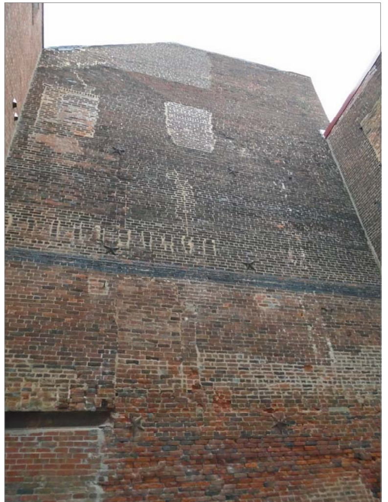
VIEW OF EAST WALL FROM REAR YARD (100 PRINCE STREET)
