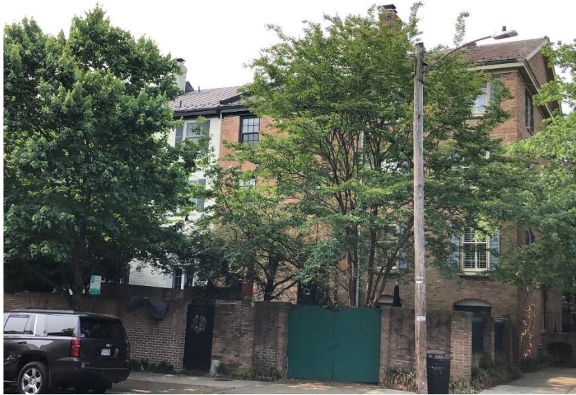
Figure 1: 422 Princess is third from right, lighter color. Notice that the other two roofs are shingled.
