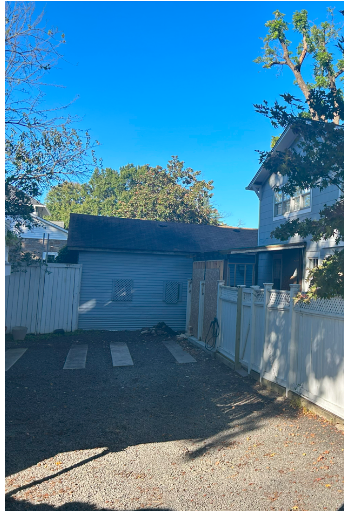
VIEW OF SHED FROM 1400 MOUNT VERNON AVE DRIVEWAY
