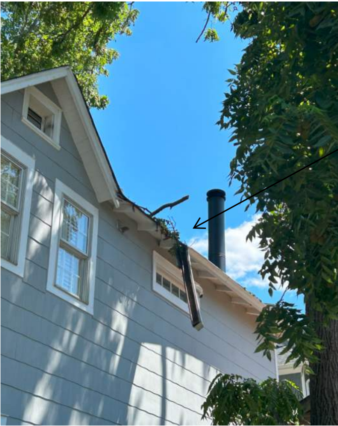
Climbing rose blown off shed wall, causing it to pull away from structure, requiring replacement
