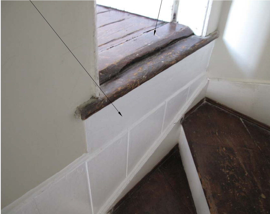
23" STEP FROM WINDERS TO THIRD FLOOR REAR BEDROOM
