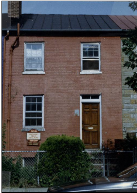
1990 Photo of Original Windows and Transom
