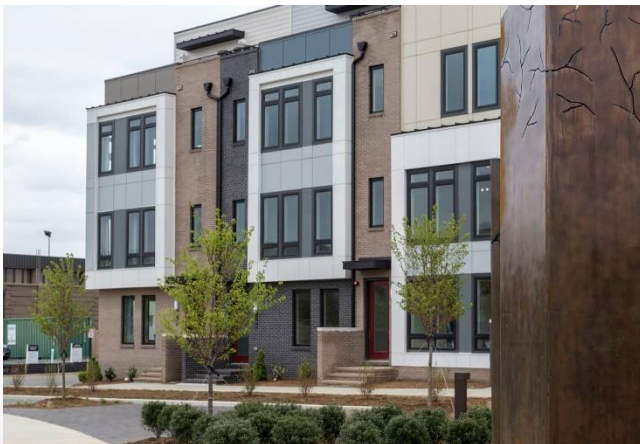
2901 Eisenhower Avenue - Central Alexandria
