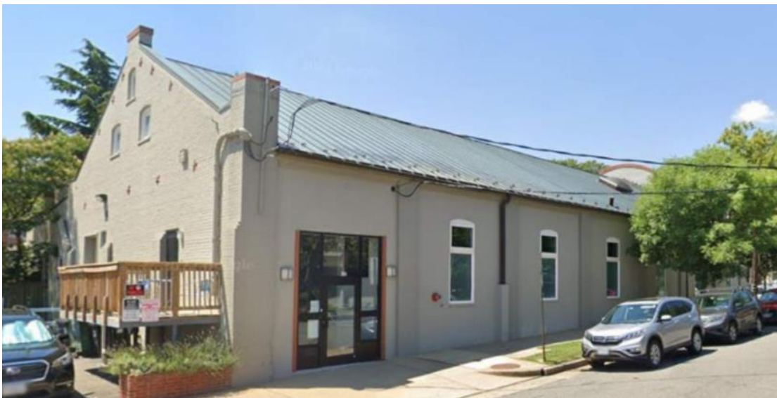
Figure 1: View of building and area of proposed dormer from Queen Street
