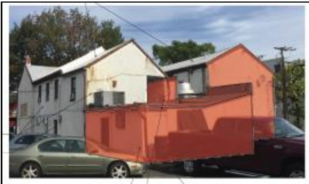
Figure 1: Area of demolition on the south (rear)
