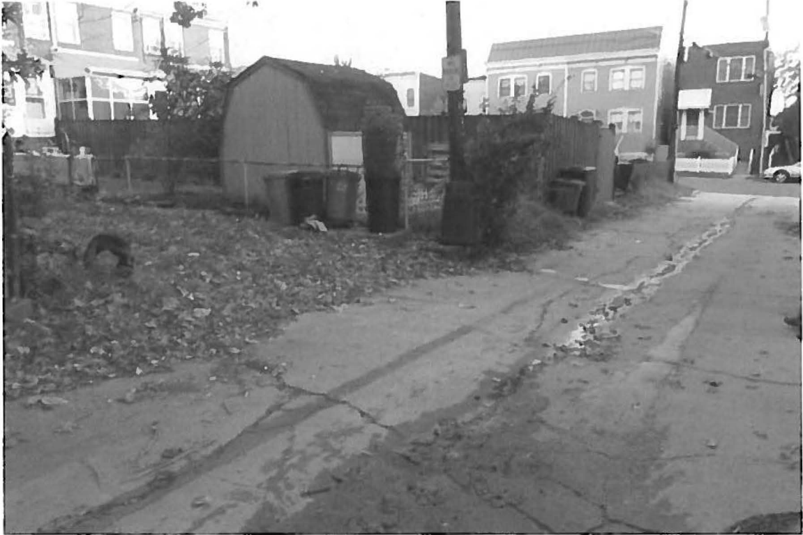
view of backyard entrance and alley
