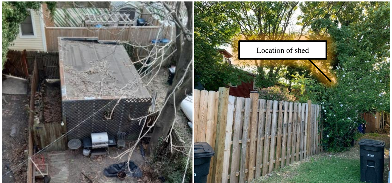
Figure 2a (left) shows an aerial view of the existing shed. Figure 2b (right) shows the visibility of the shed while standing in the public alley to the southwest of the subject property.
