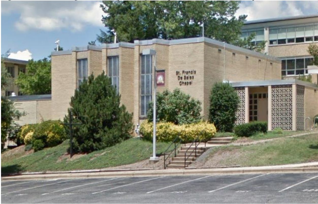
Figure#2: View looking northwest of existing Bishop Ireton High School Chapel
