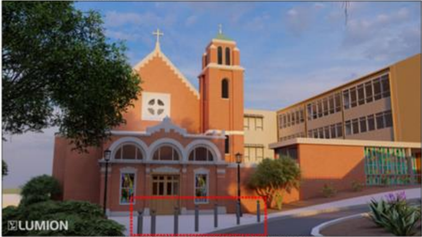
1 M-1 NTS VIEW LOOKING AT FRONT/EAST ENTRANCE
