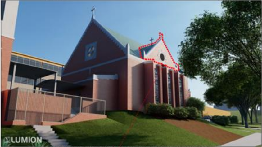
1 M-1 NTS VIEW LOOKING AT SOUTH AND WEST ELEVATIONS
