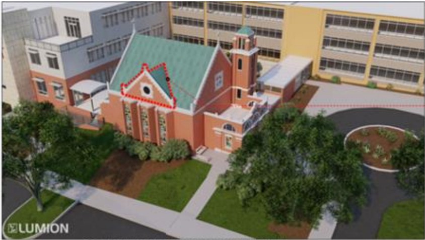
1 M-1 NTS AERIAL VIEW LOOKING NORTH WEST
