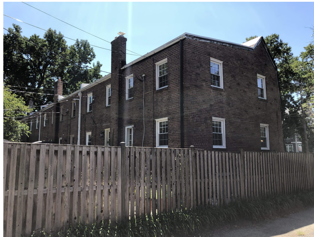
4. 1403 TO 1411 MT. VERNON AVE. REAR FACADES
