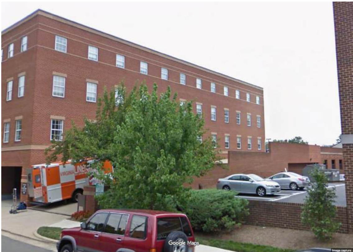
Southern Façade of Building at Garage Ramp as seen from Fairfax Street
