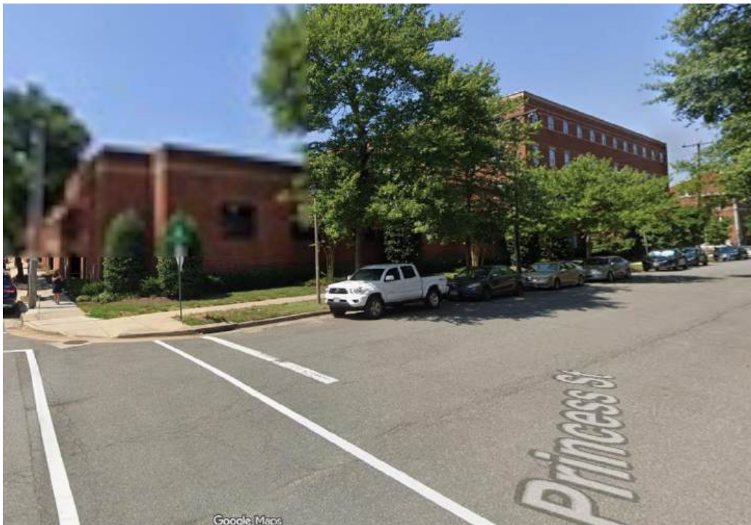
Northern Façade of Parking Garage and Building as seen near intx. of Lee Street
