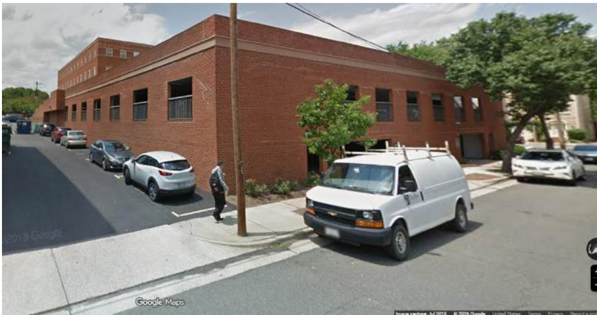
Eastern and Southern Facades of Parking Garage as seen from Lee Street alley entrance
