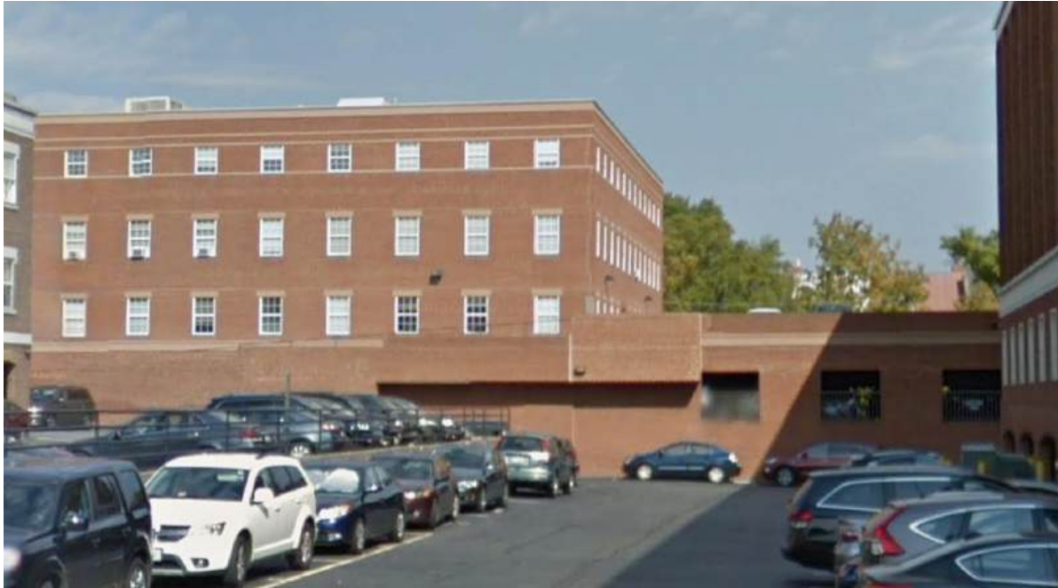
Southern Façade of Building and partial view of garage as seen from Queen St.
