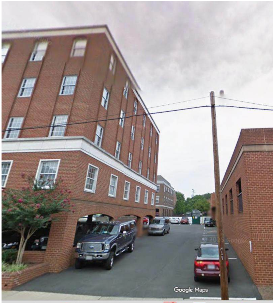
Northern Façade as seen from alley entrance on Lee St. near intx. with Quay St.
