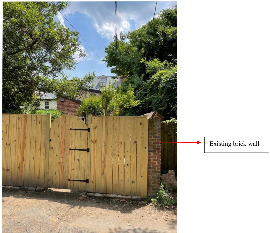
Figure 2 - Existing rear wood fence to be replaced
