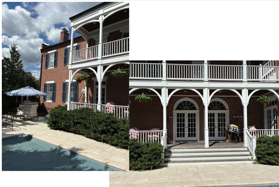
EXISTING PHOTOS AT EXISTING EAST WALL
