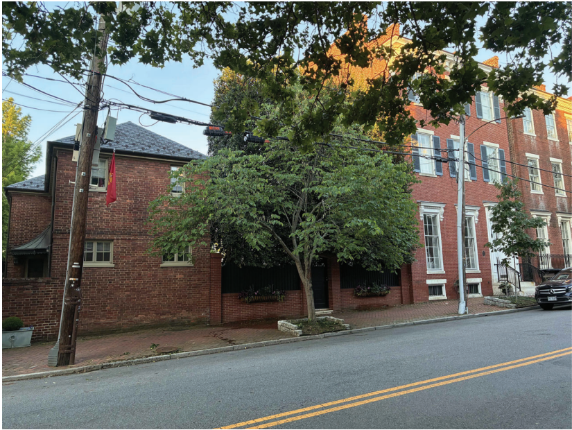
EXISTING FROM (NORTHEAST) ON DUKE STREET
