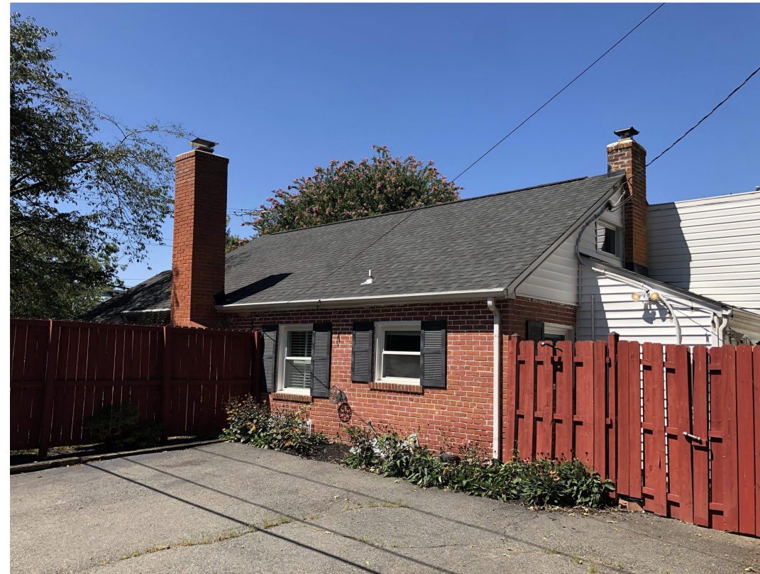
2. 1413 MT. VERNON AVE SIDE AND REAR FACADE
