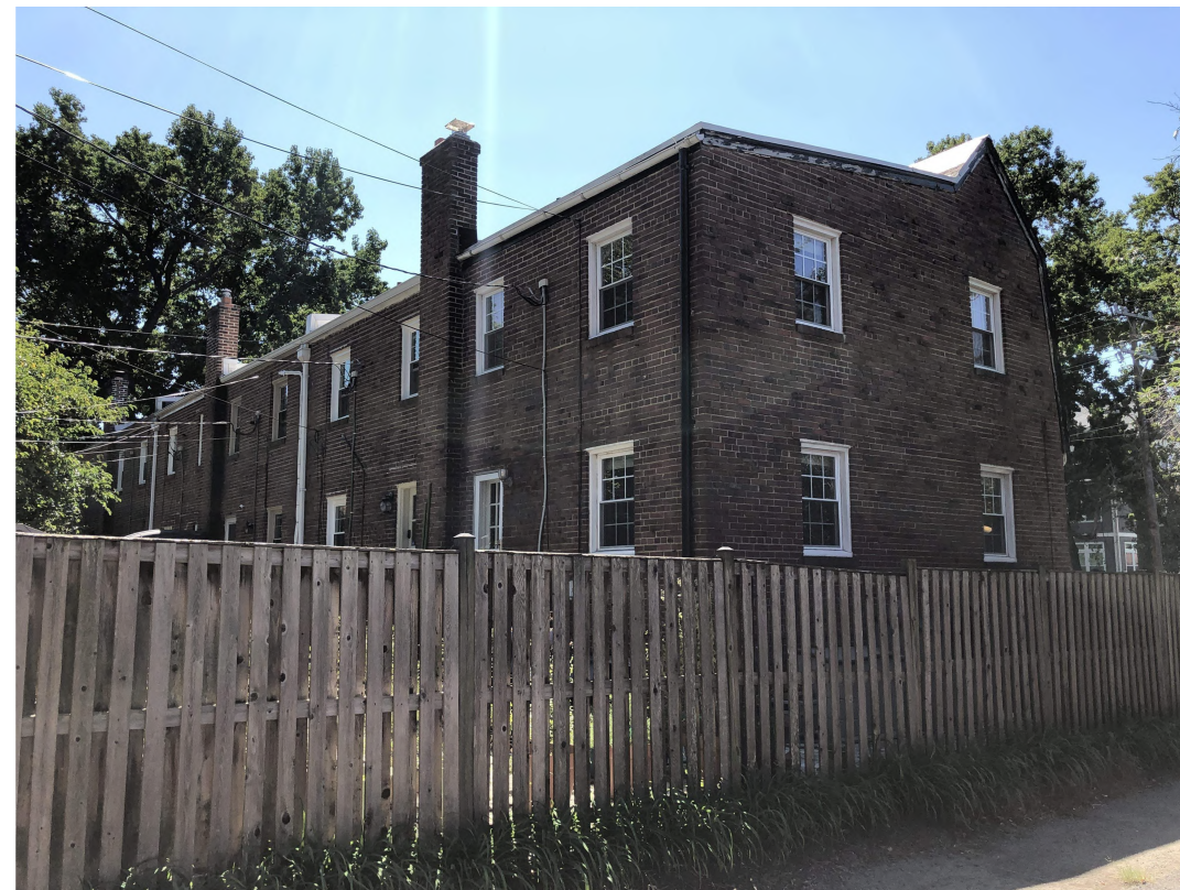
4. 1403 TO 1411 MT. VERNON AVE. REAR FACADES
