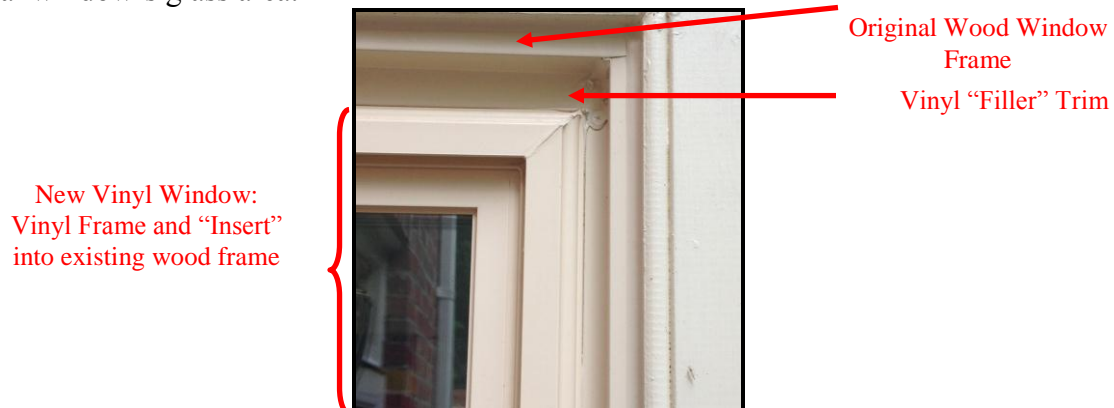
Figure 5: Detail of Installed Vinyl Insert Window
