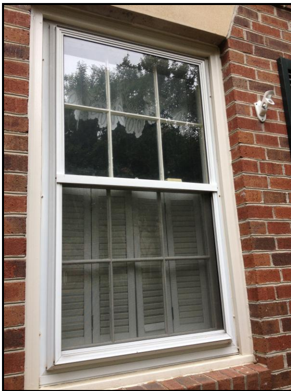
Figure 1: Photo of Original Wood Windows with Storm (on neighboring Property)
