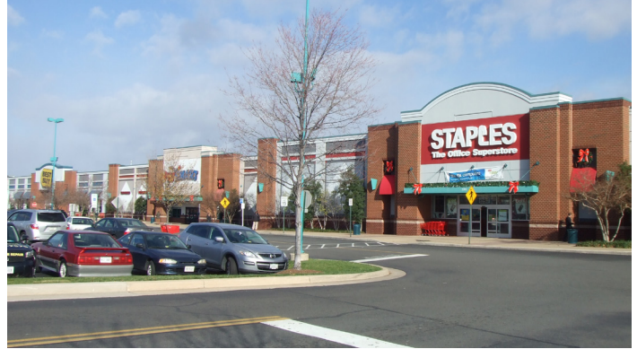
Existing Potomac Yard Shopping Center
