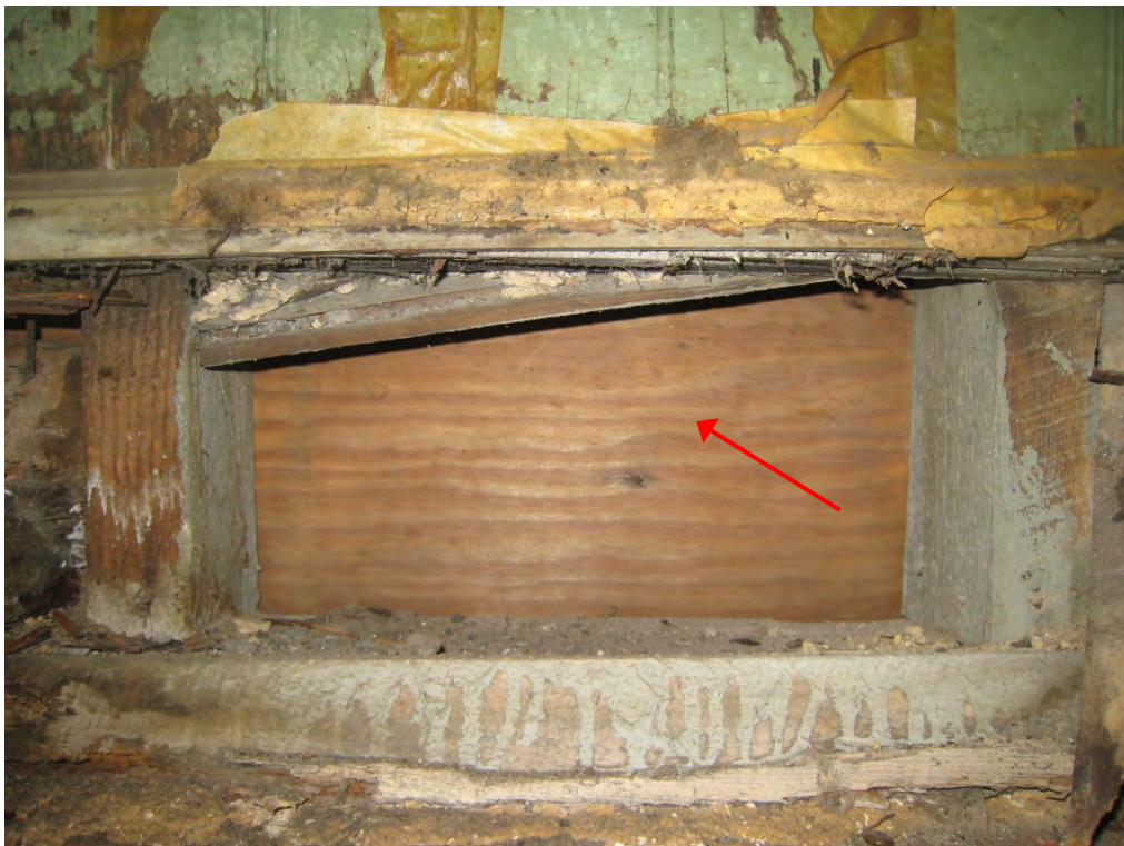
Figure 6 – View from interior of existing rear “el” addition of plywood sheathing on exterior studs
