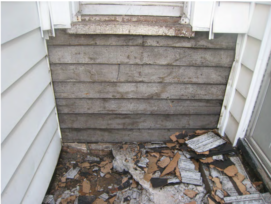
Figure 4 – Wood siding on east elevation of main house block visible after removal of aluminum and asphalt siding
