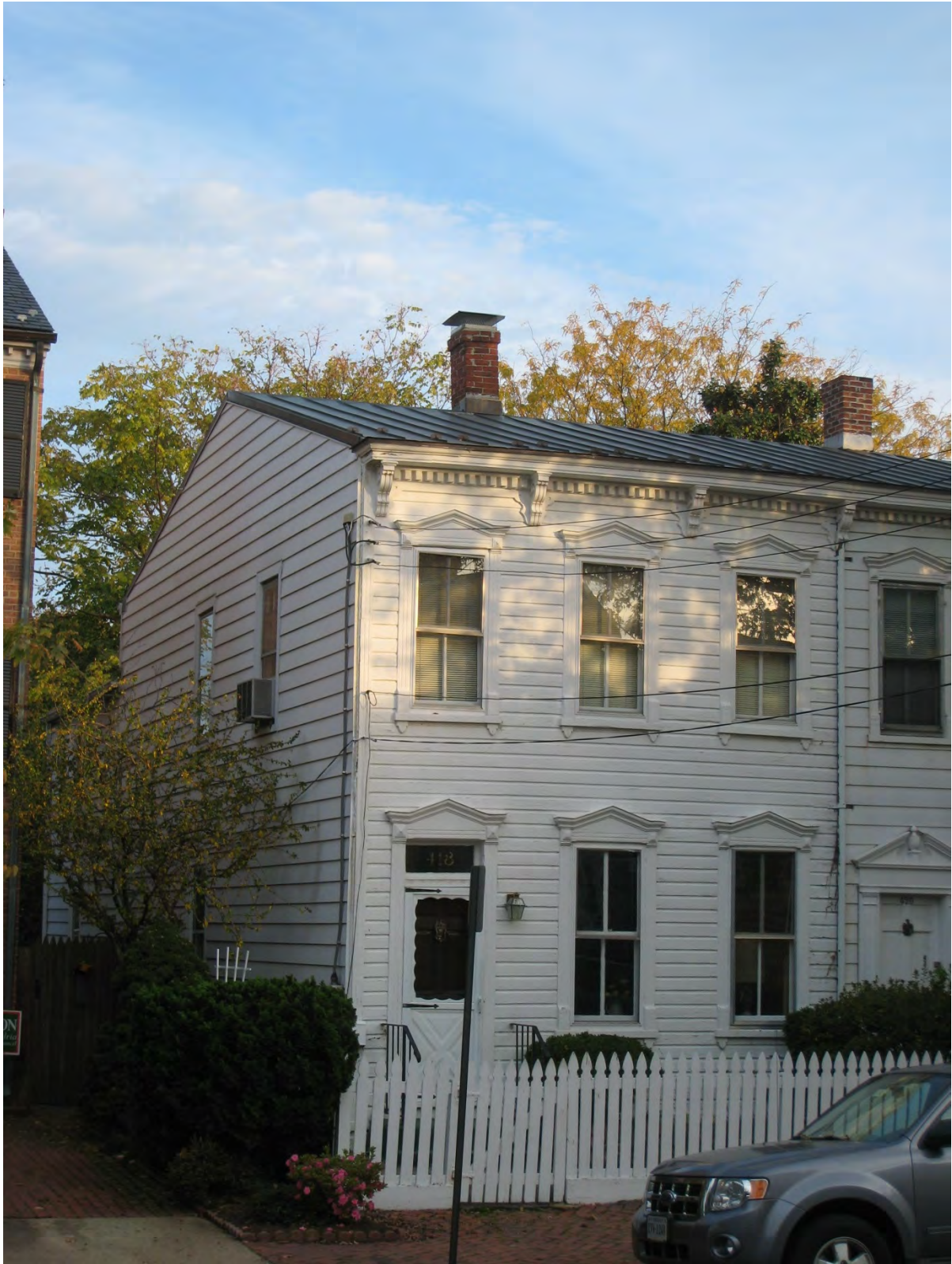
Figure 2 – View of main block looking east
