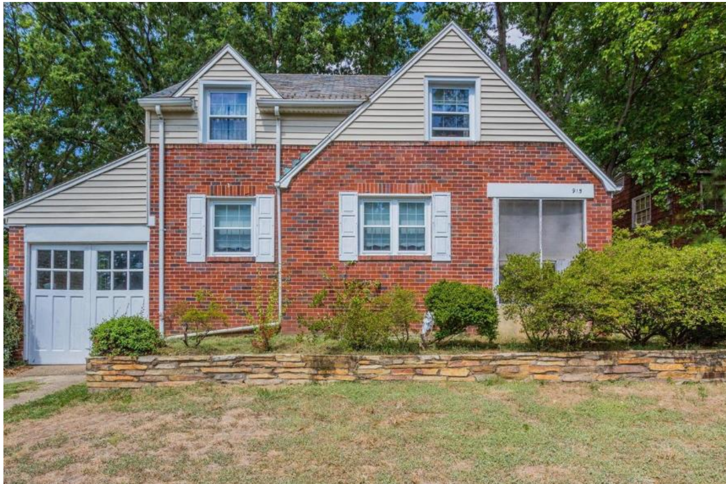
Existing dwelling to be demolished
