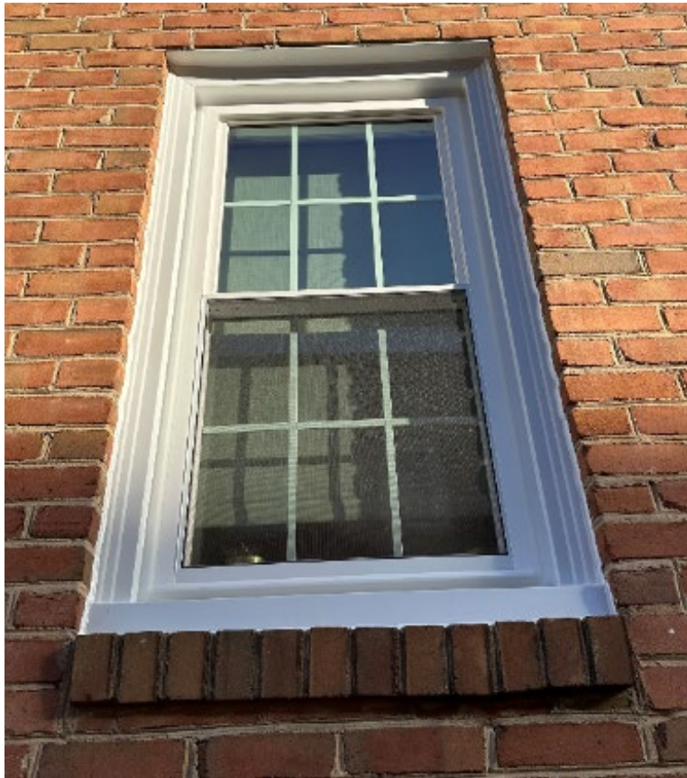
Figure 2: Installed vinyl window with sandwich muntins
