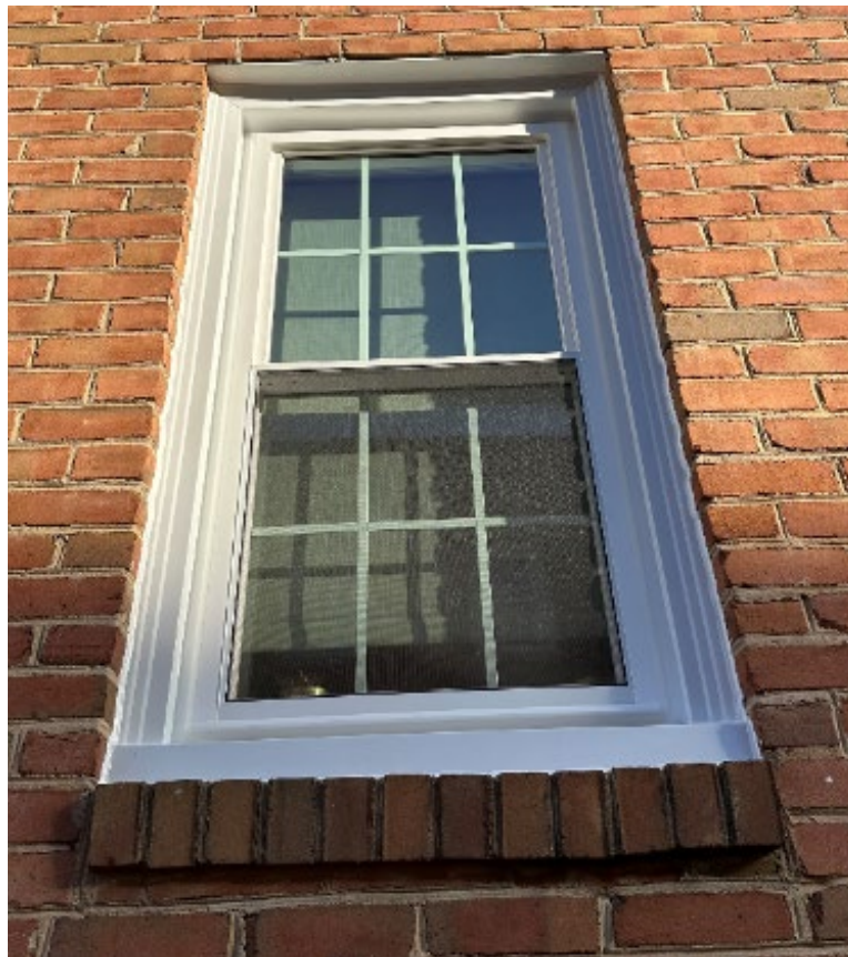
Figure 2: Installed vinyl window with sandwich muntins
