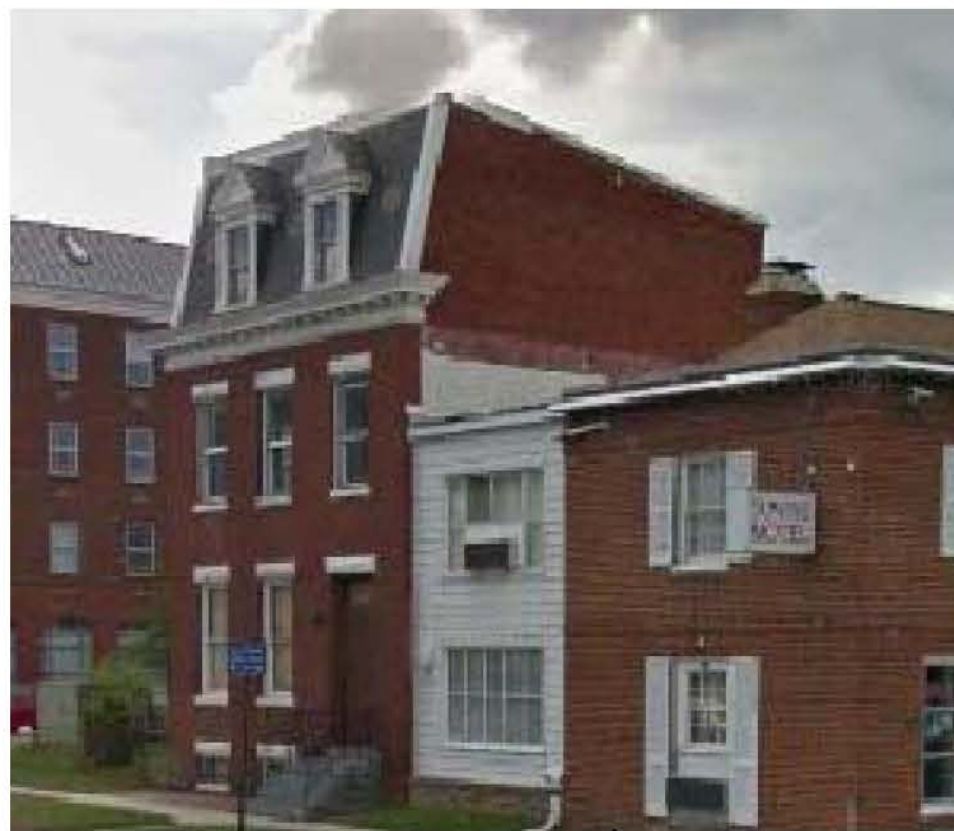
EXISTING BUILDING WITH NEWLY EXPOSED BRICK PARTY WALL
