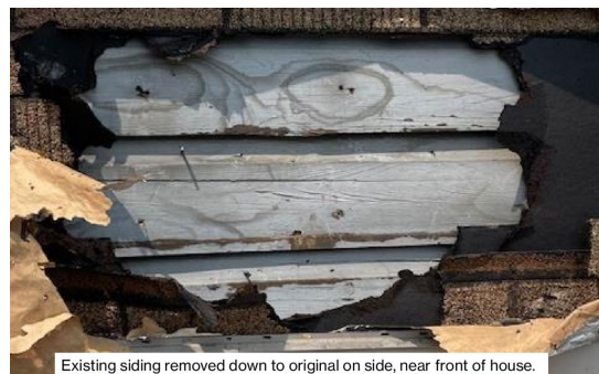
Figure 4: Portion of siding removed to expose original siding
