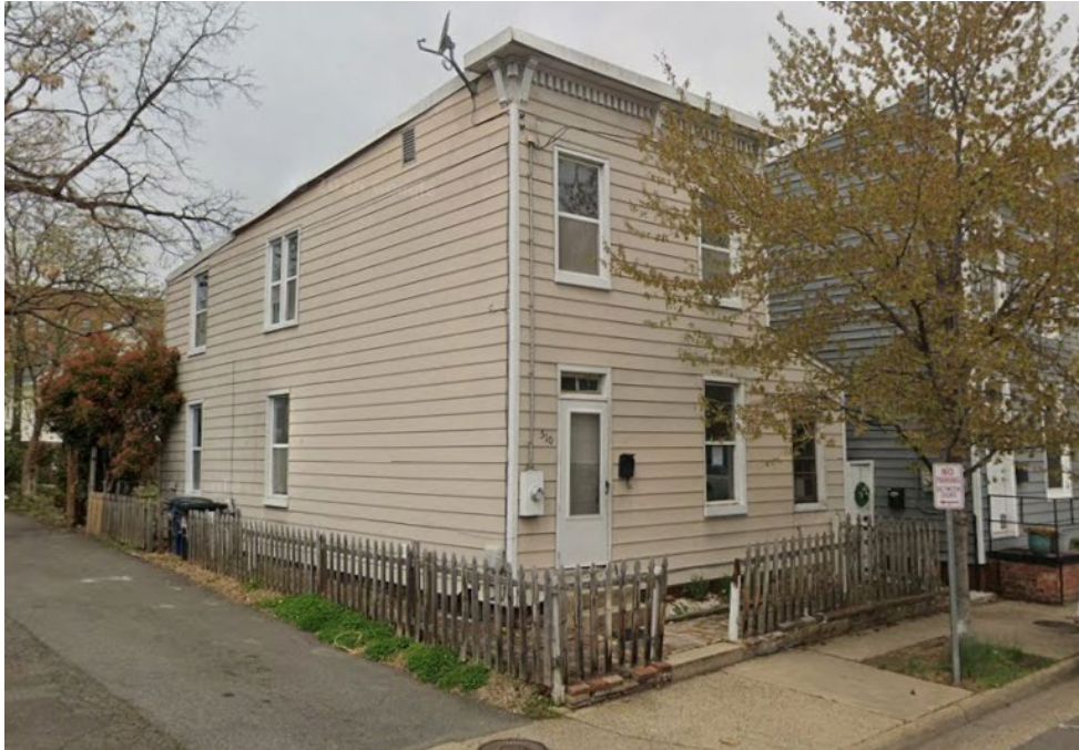
Figure 1: View of 510 N Patrick Street with modified second floor window and ground floor addition
