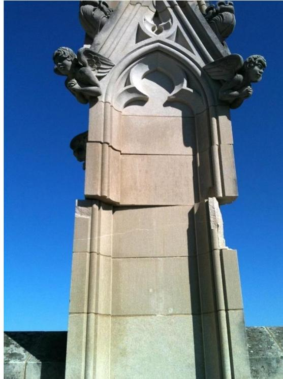
**Figure 26: Earthquake Damage to Washington National Cathedral in Washington, D.C. After the 2011 Earthquake<sup>78</sup>**
