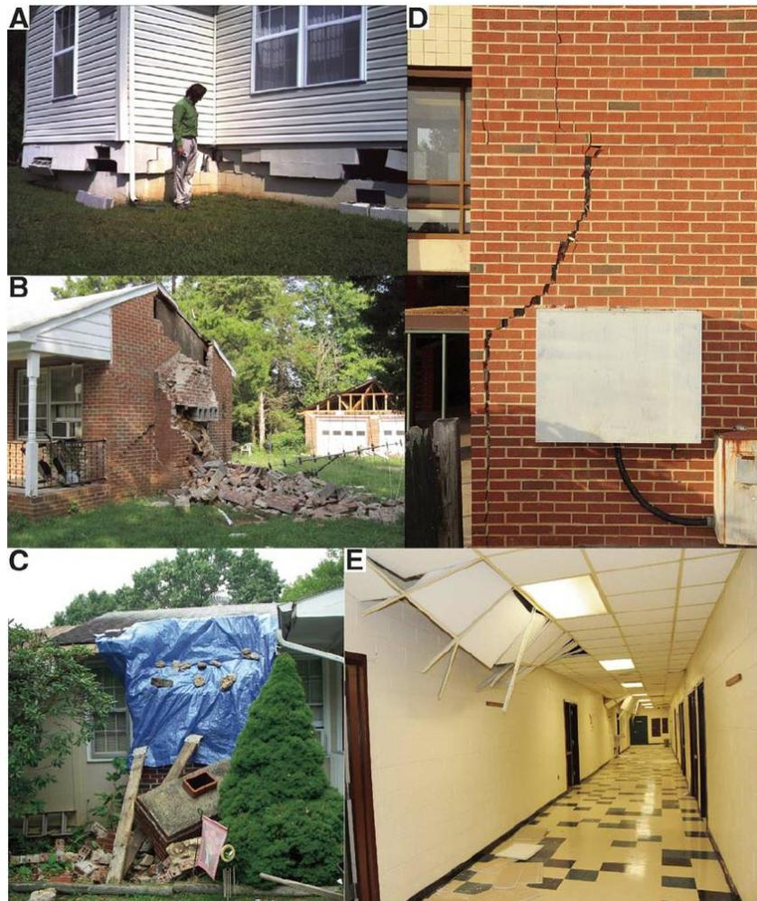
**Figure 25: Examples of Structure Damage in Louisa County, Virginia After the 2011 Earthquake<sup>77</sup>**
