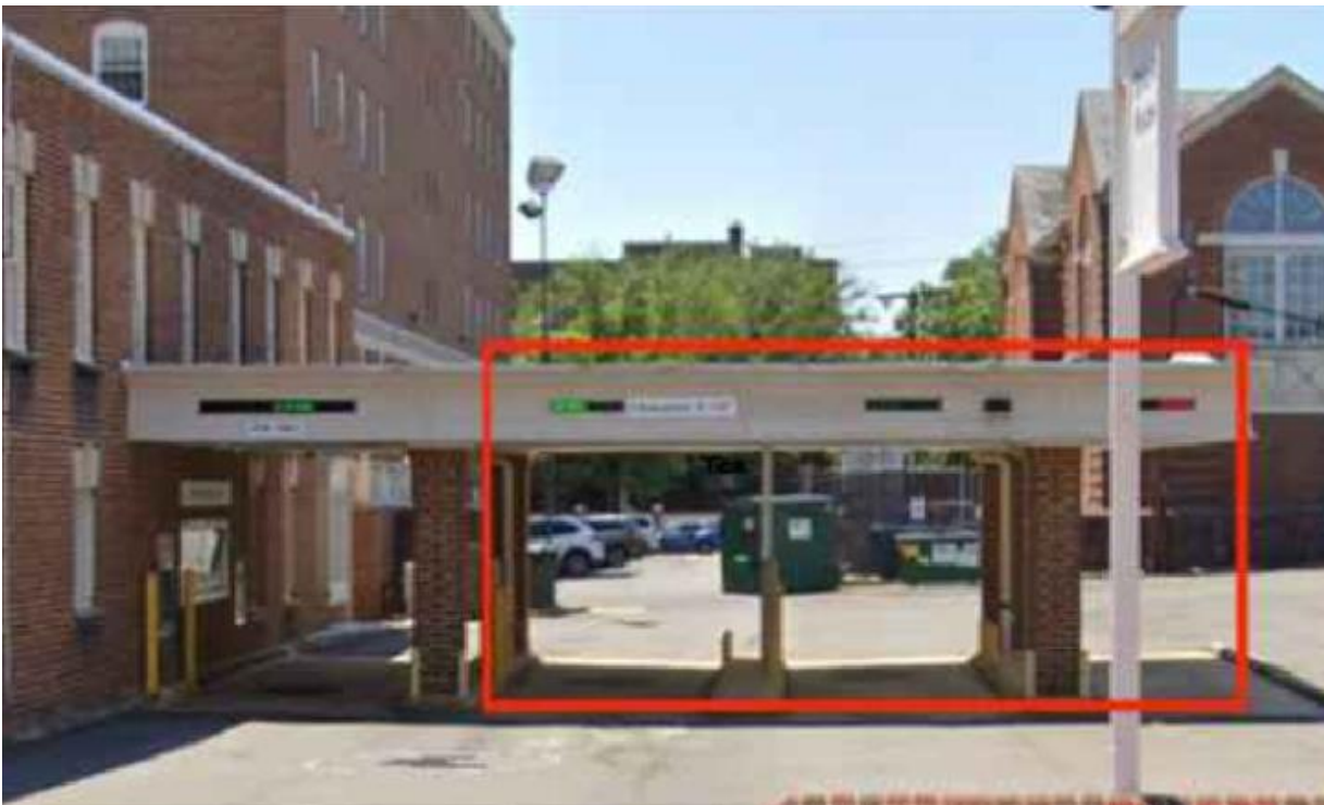
Figure 1: Extent of canopy to be demolished
