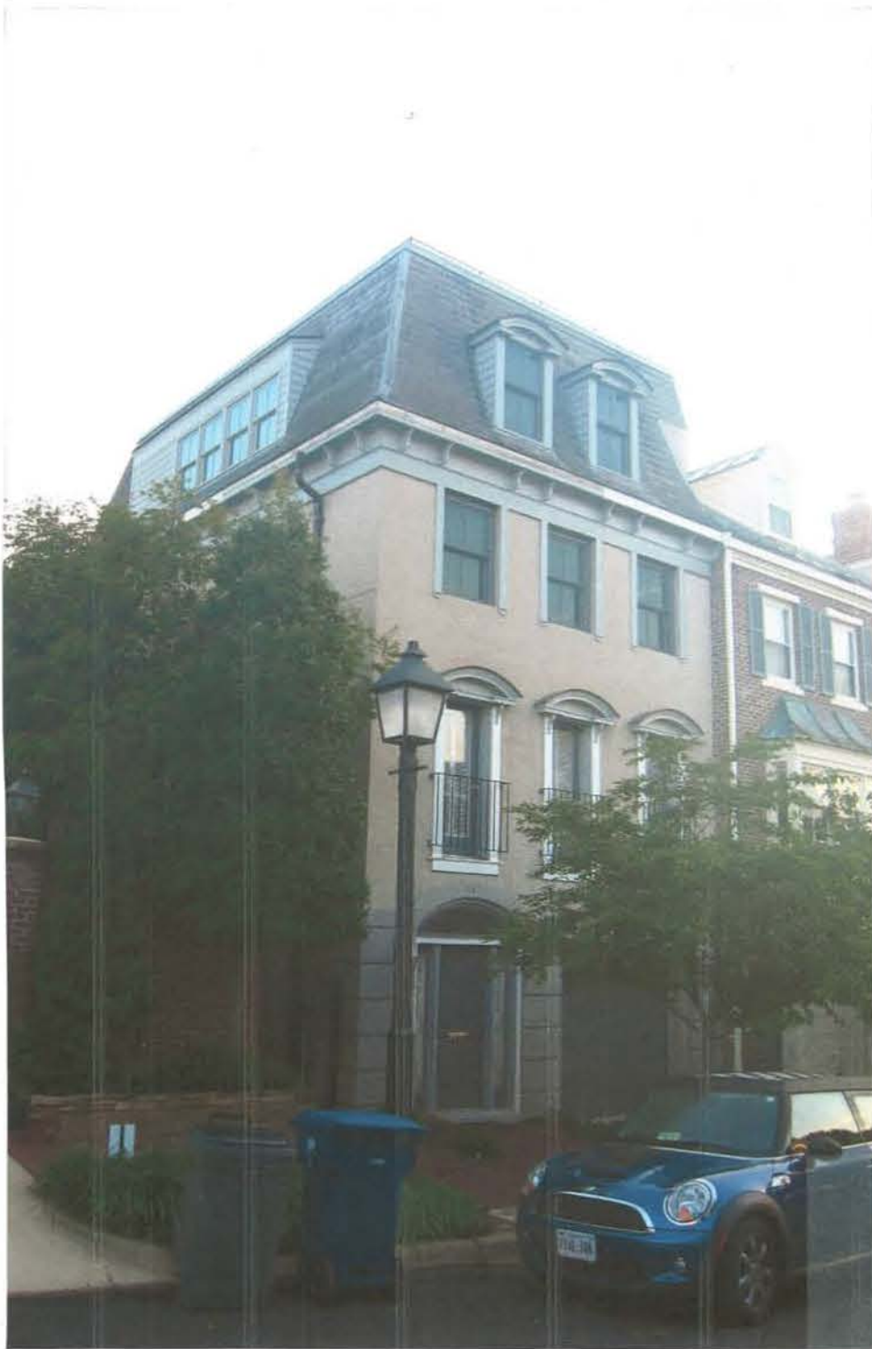
Townhouse on Wolfe in same Waterford development w/ Mansard Roof & full attic storage
