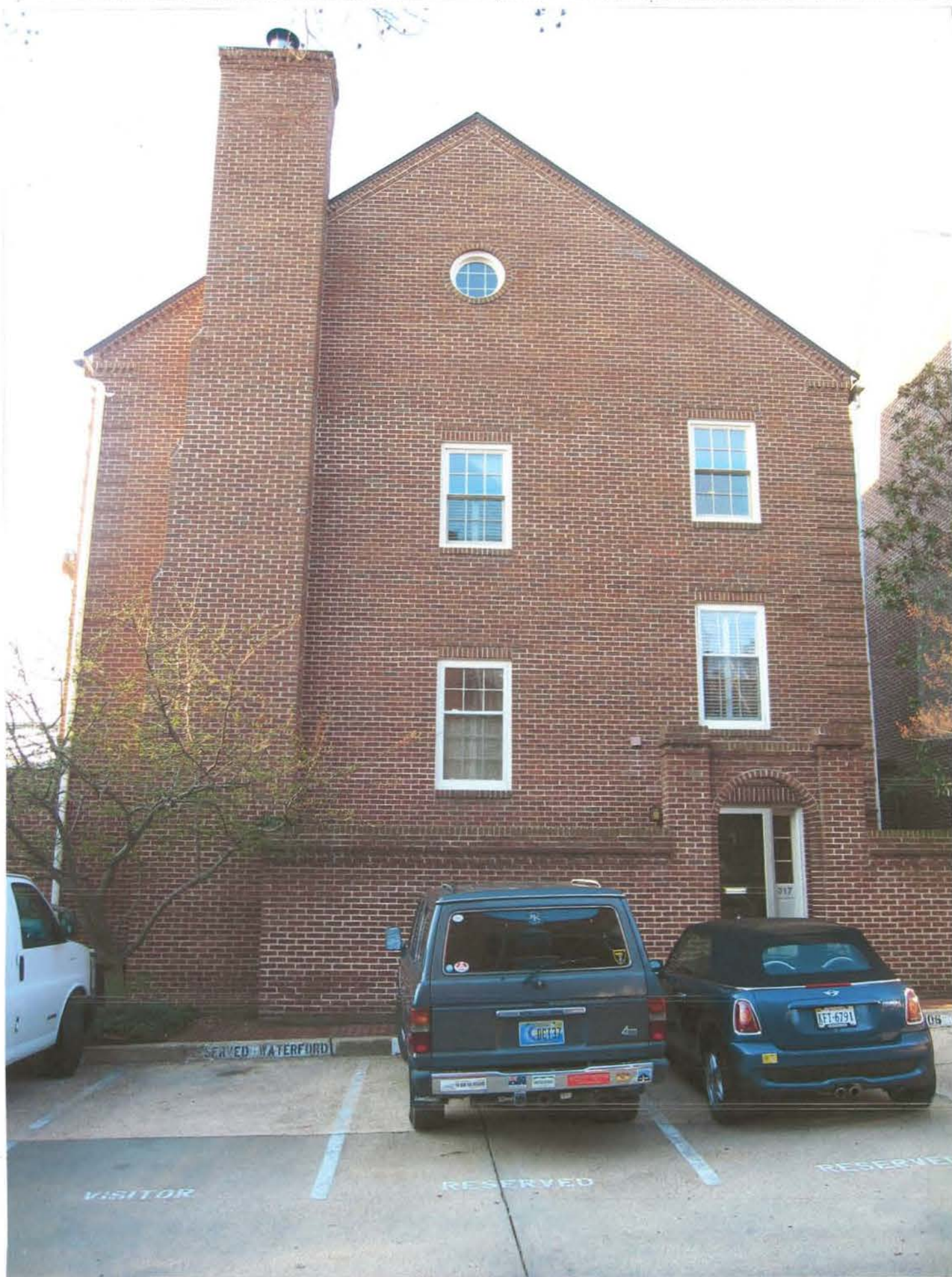
Existing West Side of 317
