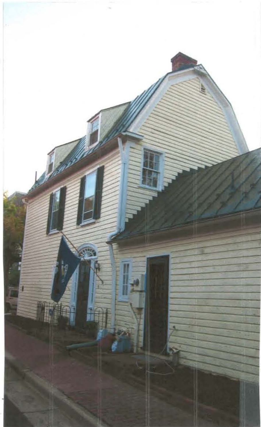
Gambrel roof at Wolfe & Potomac Court (historic)
