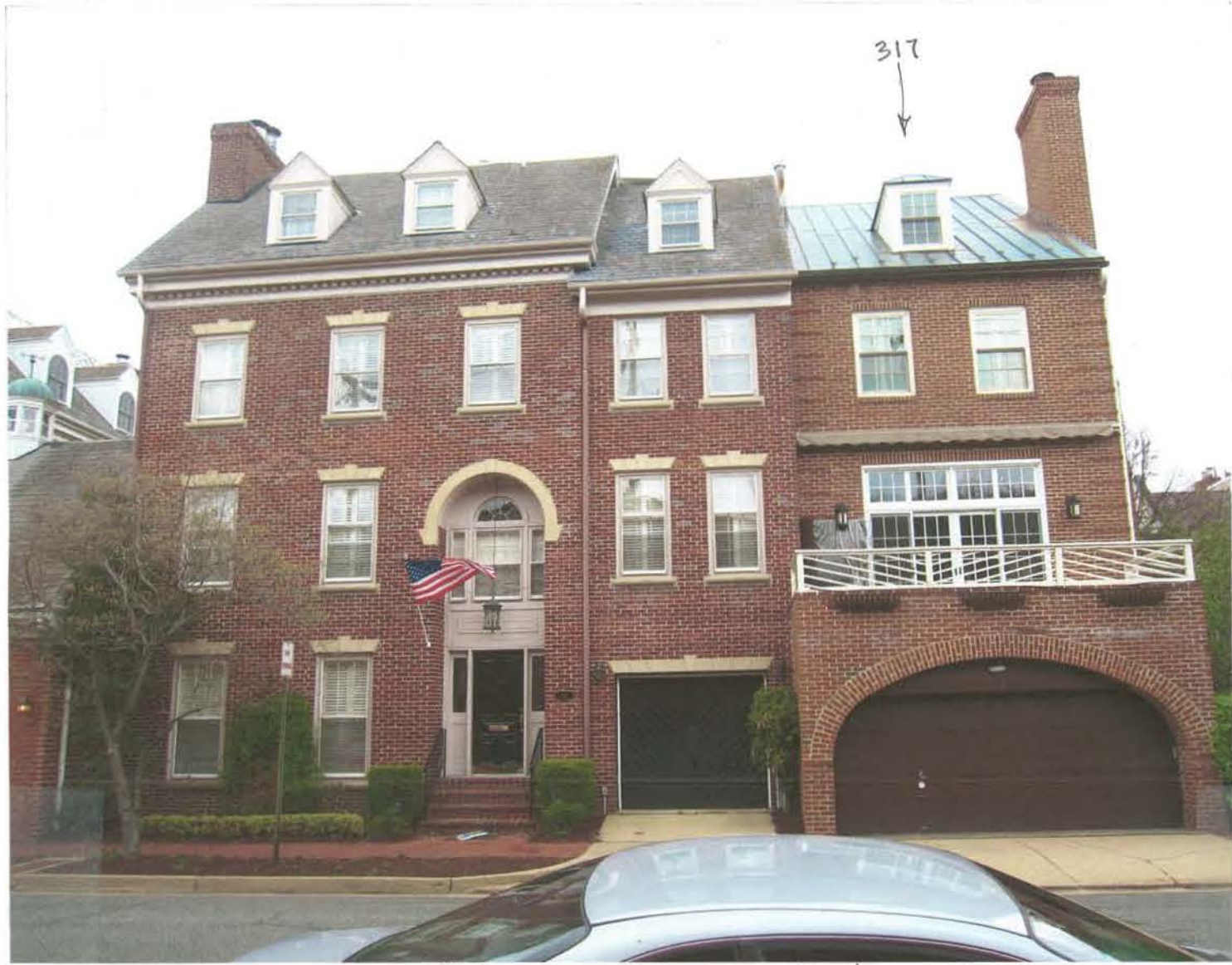
East Face of 319 & 317 S Union Street
