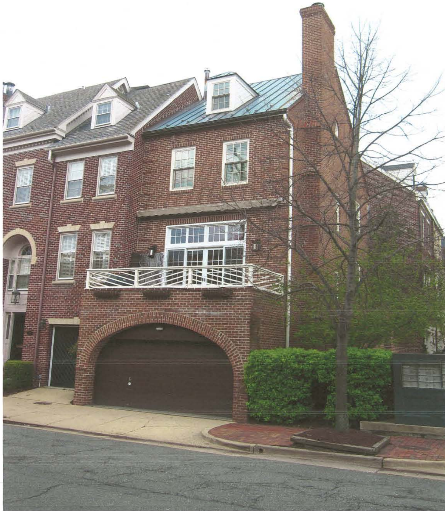
Existing Front at 317 S. Union
