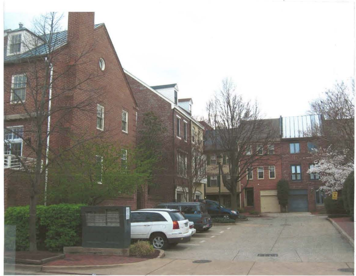
Existing North Side of 317 S Union and Neighboring Properties
