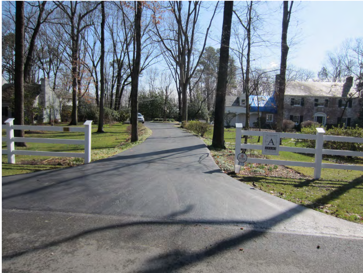
915 Vicar Lane Existing Driveway Entrance and Front of House
