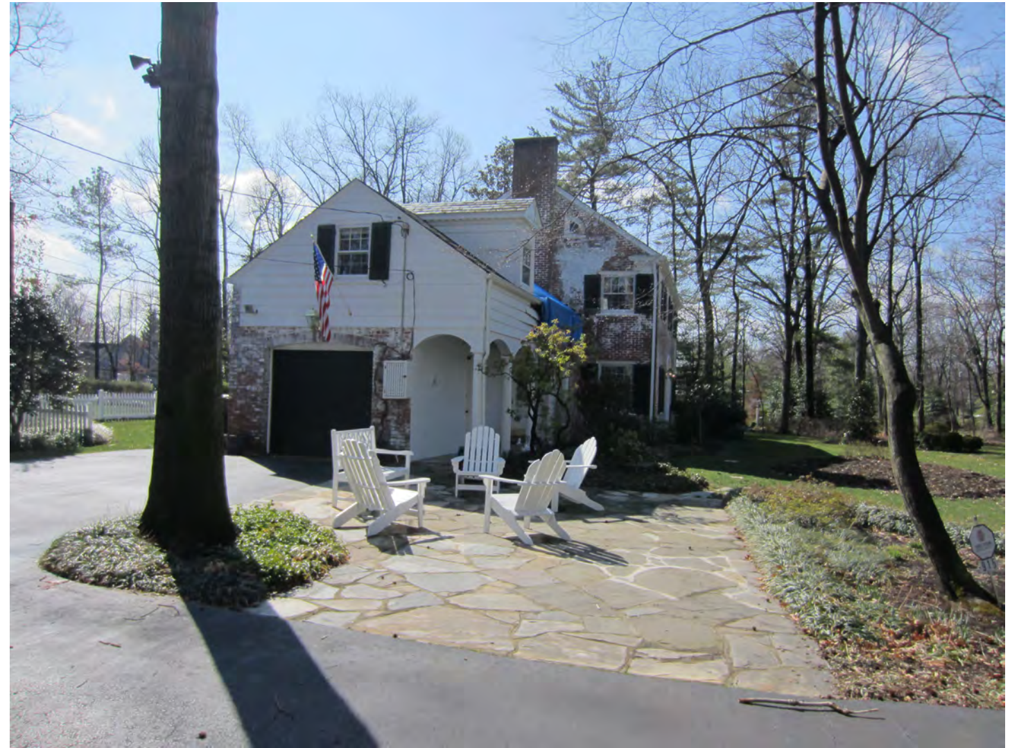
915 Vicar Lane Existing Garage Wing
