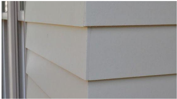
TYPICAL SIDING James Hardie painted fiber cement lap siding with 3" exposure. Biscuit siding edges for mitered corners, no corner board trim.
