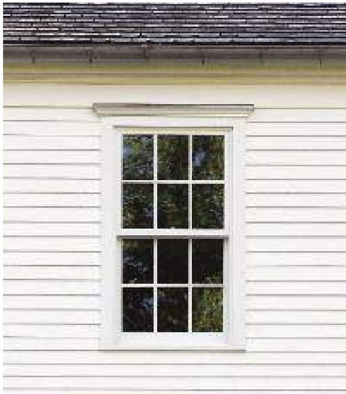
NEW EXTERIOR WINDOWS New windows to be Windsor painted wood SDL w/ muntins to match existing profiles, insulated glass, white jamb liners and screens with oil rubbed bronze hardware.
