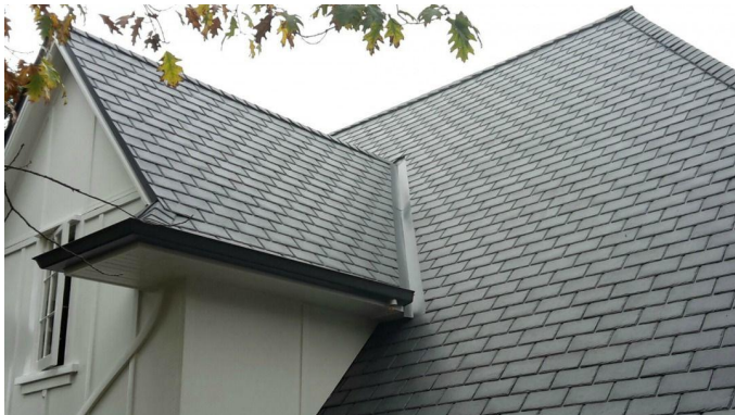
SHINGLE ROOF Synthetic slate shingle roof by Ecostar on new roof framing.
