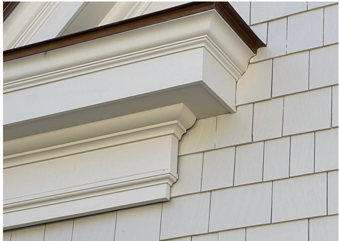
EXTERIOR TRIM Ptd Boral at all ptd. trim locations - includes window/door casing; bandboards; roof eave, fascia and rake moulding
