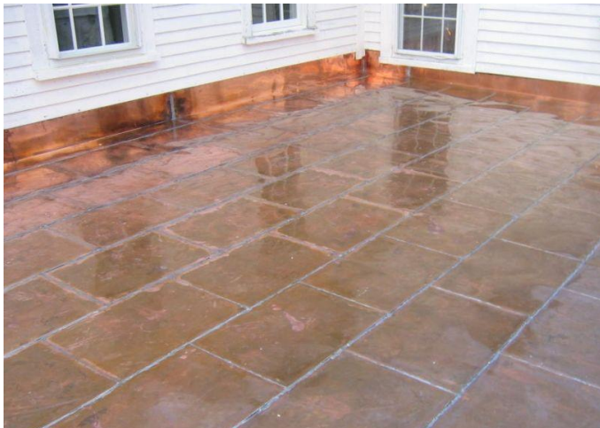
METAL ROOF Flat seam copper roof at new entry portico
