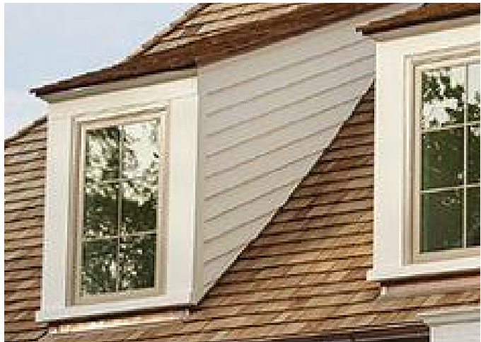
DORMER & GABLE ROOF SIDING Painted V-groove PVC panels as shown on elevations. At dormers, siding is oriented, so it runs parallel to main roof slope.
