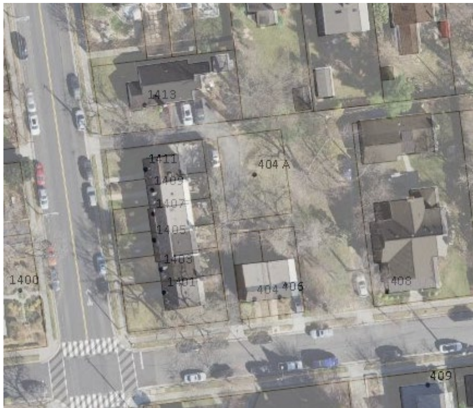
Figure 7 – Aerial showing orientation of existing buildings
