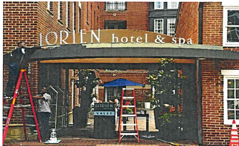
EXISTING SIGN TO BE REMOVED & REPLACED
