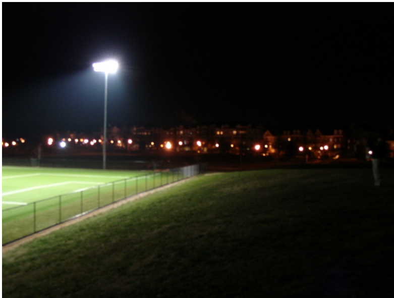
Comparable examples of sports' facility lighting luminaires: Ben Brenman Park – note the lights are mounted on 70 ft. poles.
