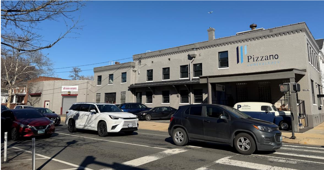
Figure 1: View of existing building from North Henry Street
