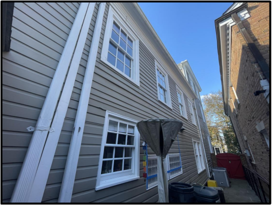
AREA OF WORK - FIRST FLOOR DOUBLE-HUNG AND GLASS BLOCK WINDOWS TO BE REMOVED; BLUE TAPE INDICATES PROPOSED NEW WINDOW UNIT
