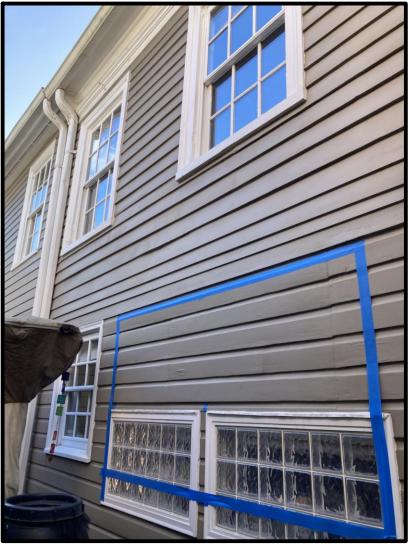
AREA OF WORK - FIRST FLOOR DOUBLE-HUNG AND GLASS BLOCK WINDOWS TO BE REMOVED; BLUE TAPE INDICATES PROPOSED NEW WINDOW UNIT
