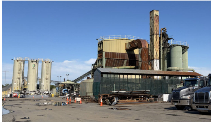
Figure 1: Virginia Paving asphalt production facility
