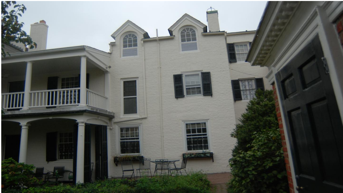
East Elevation at Area of Proposed Addition
