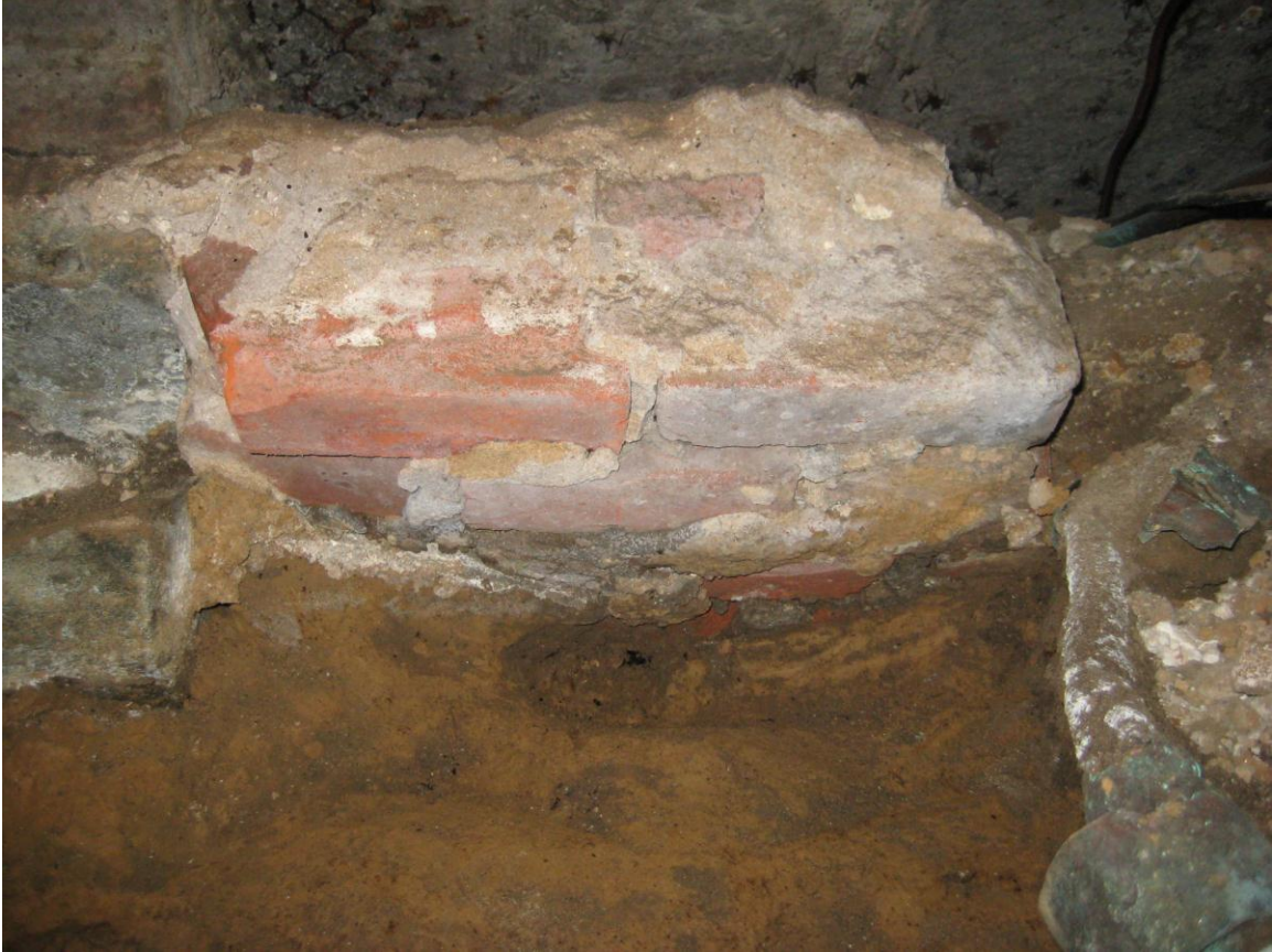
Figure 6. Detail of the two-brick-wide arch, bonded into the stone fireplace base. The area to the right of the arch has been disturbed by later construction.
