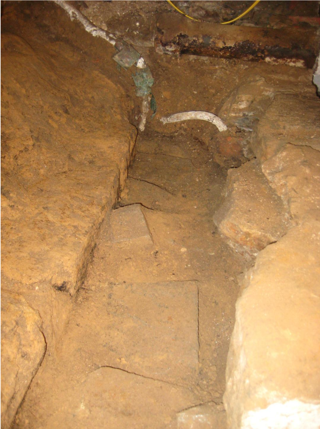
Figure 7. Detail showing the relationship of the natural clay subsoil, the builder's trench comprised of mixed sandy clay and stone, and the top of the north cellar wall after the top courses were removed. The iron drain pipe and a defunct lead water line are visible in the background.
